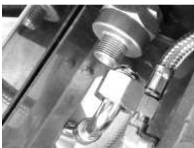
Connecting the metal hose
