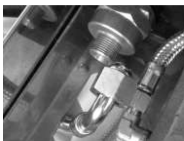
Connecting the metal hose
